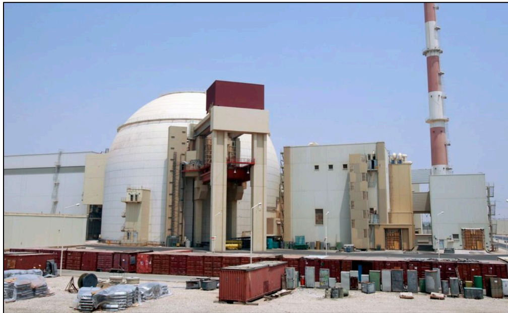
Bushehr Nuclear Power Plant. Source: Reuters
